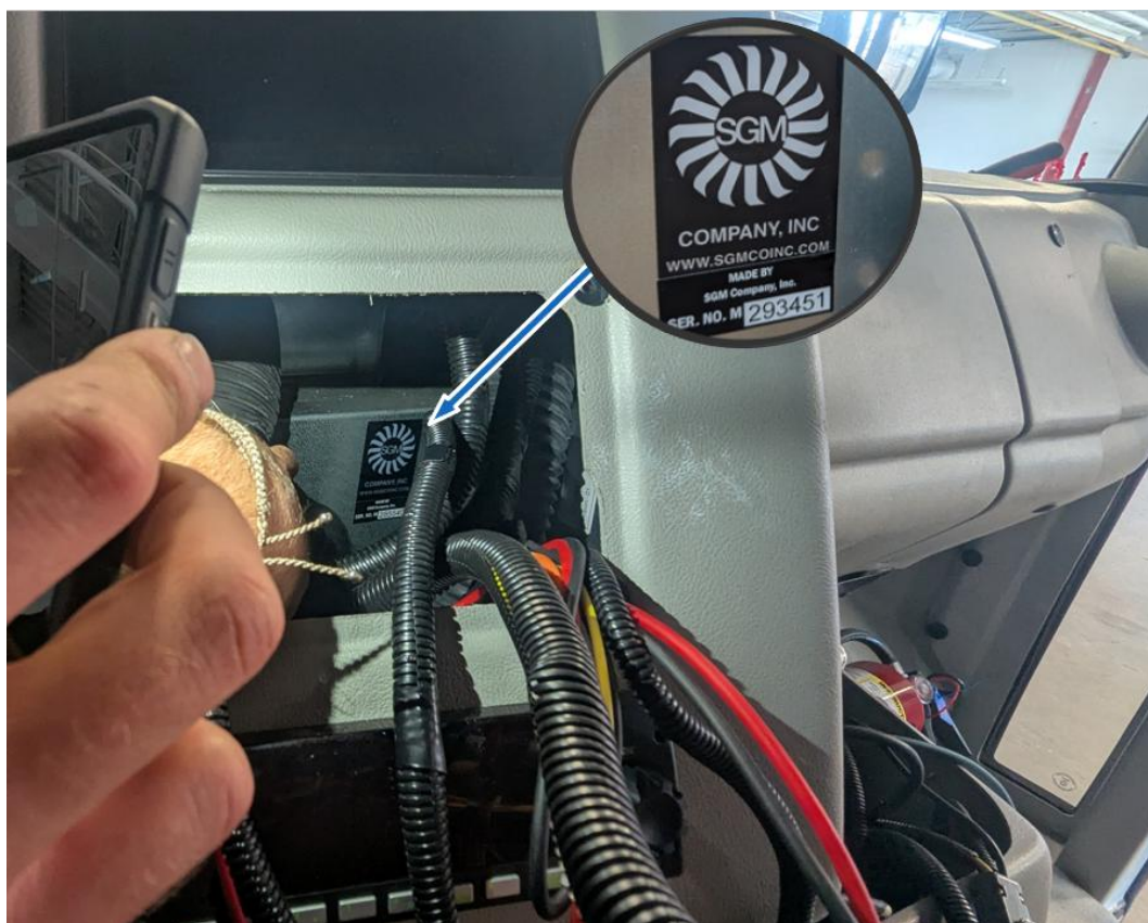
Figure 23 – Serial number of the HVAC unit
